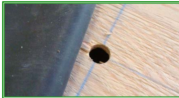
View of Prepared Plywood Deck
